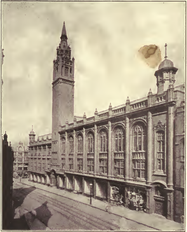
CENTRAL MISSION HALL, BIRMINGHAM
